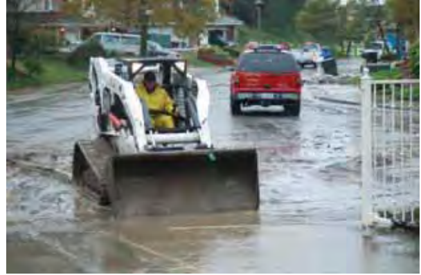
Dozer clearing mud off the street following the rains that hit the fire consumed areas of Yorba Linda.
