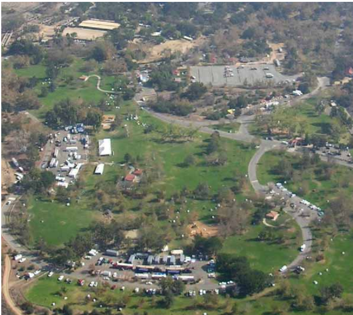
The Facilities Unit on the Freeway Complex Fire created an efficient base camp to support the needs of more than 3,800 personnel.
