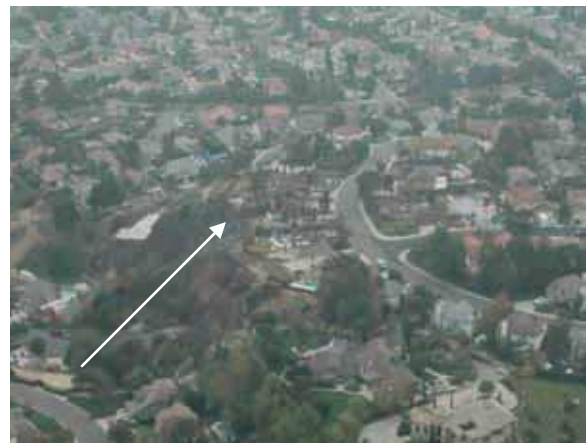
Arrow pointing to the same slope after the Freeway Complex Fire showing the tragic loss of homes along the ridge
